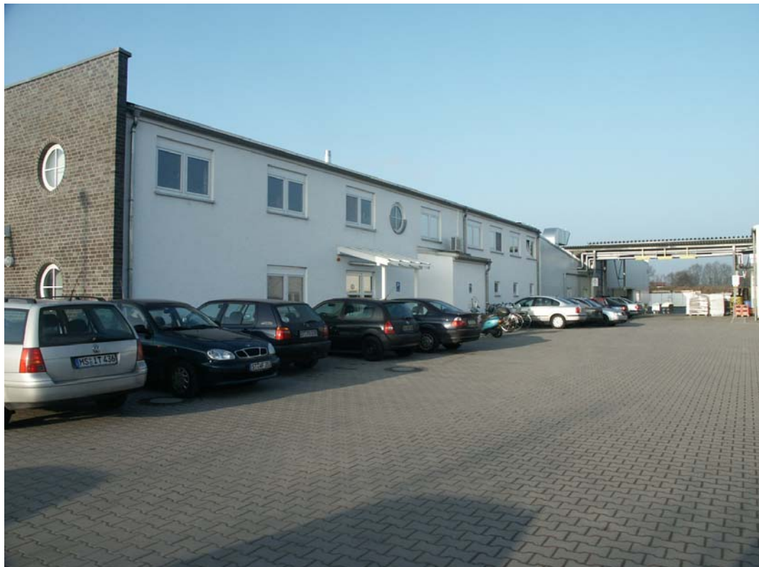
2 floors office section of the production building.
